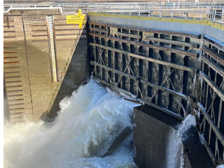
Breach Through Failed Sill
